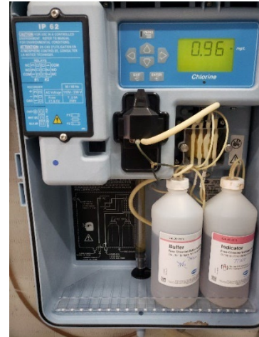
PHOTO 7.2.2 – CHLORINE ANALYZER
