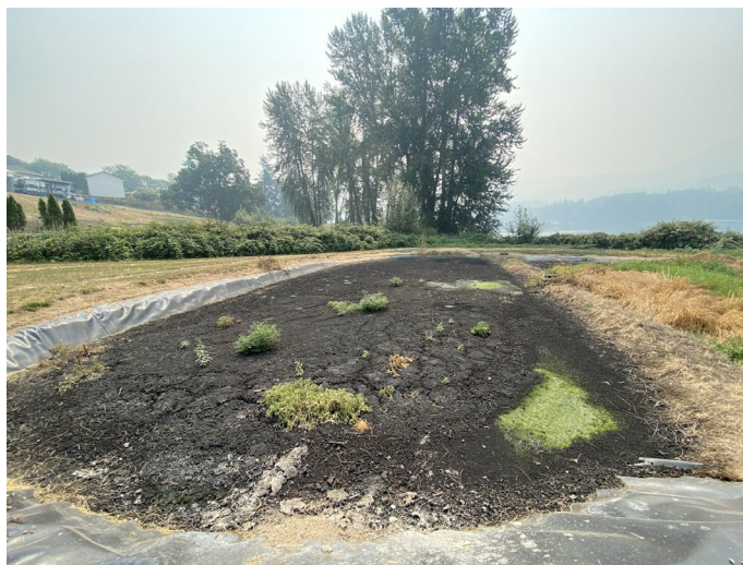
Figure 2-13: Eastern Sludge Drying Bed
