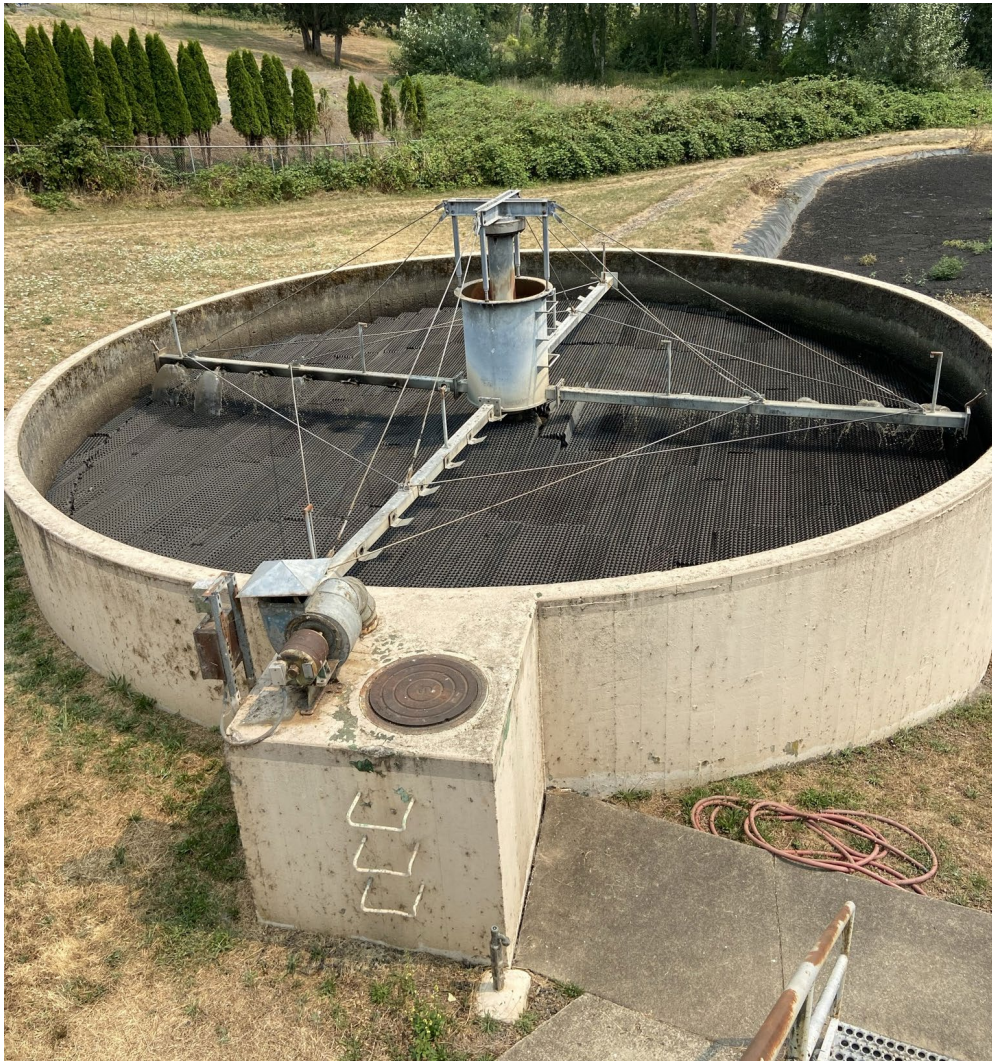
Figure 2-10: Trickling Filter with Polypropylene Media
