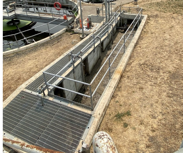
Figure 2-11: Solids Contact Channel
