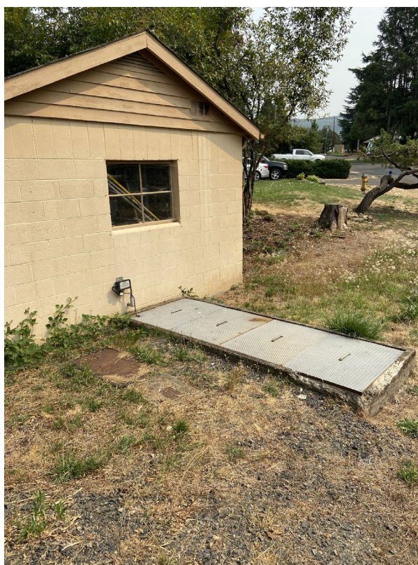
Figure 2-1: Alder Street Pump Station
