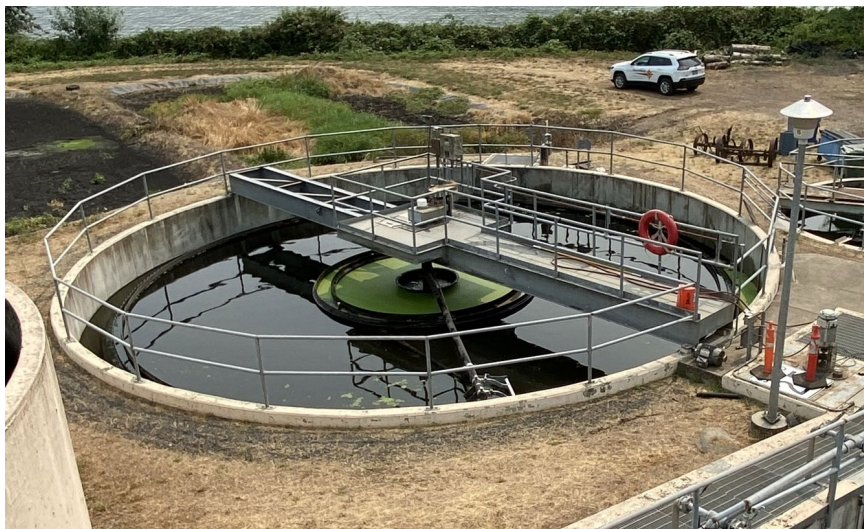
Figure 2-12: Secondary Clarifier
