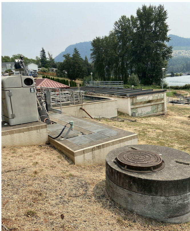
Figure 2-6: Manhole upstream of the WWTP Headworks
