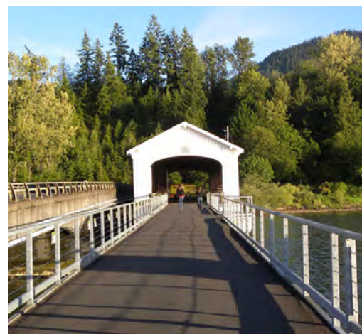
Lowell Covered Bridge Interpretive Center Source: Eugene, Cascades & Coast - Travel Lane County
