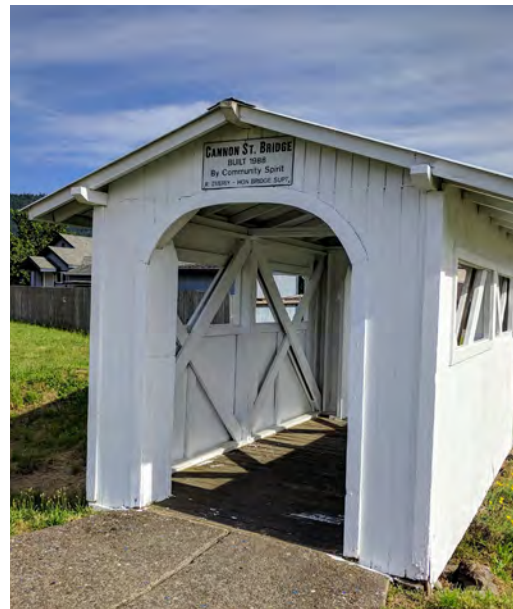
Cannon Street Bridge at Rolling Rock Park
