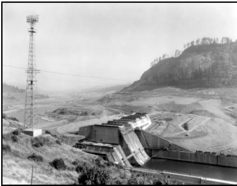
Construction of the dam at Lookout Point, 1952
