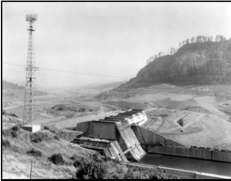
Construction of the dam at Lookout Point, 1952
