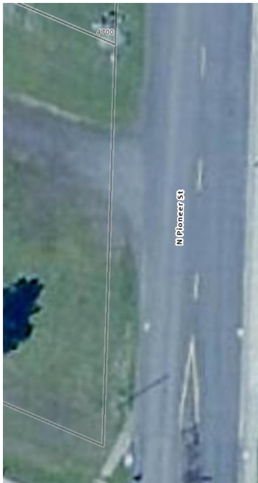
Image 4. Frontage of North Pioneer Street abutting the site. No urban street improvements currently exist.
